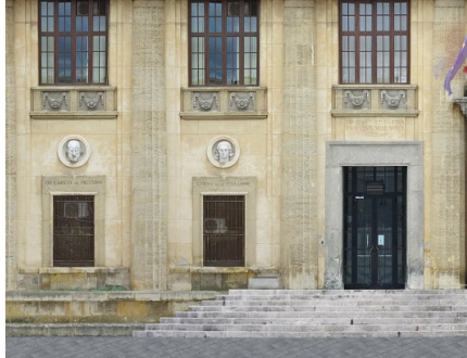
Facade orthomosaic GeoTiff (.tif)
